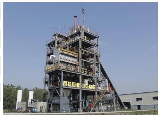
FINAL GAS CALORIFIC VALUE CAN REACH UP TO 2500KCAL/NM<sup>3</sup>
