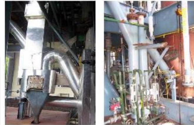
**Fly ash recycle with non mechanical valves (loop seals) to improve carbon conversion – similar to CFB boilers**
